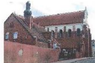
145. Bydgoska 23, mur prob.
